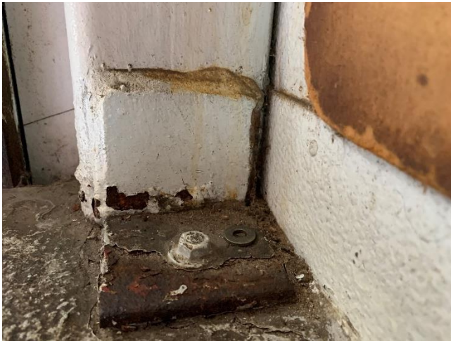
Figure 1. The angle seems to be intact, and only slight rusting is visible. (Level 1)
