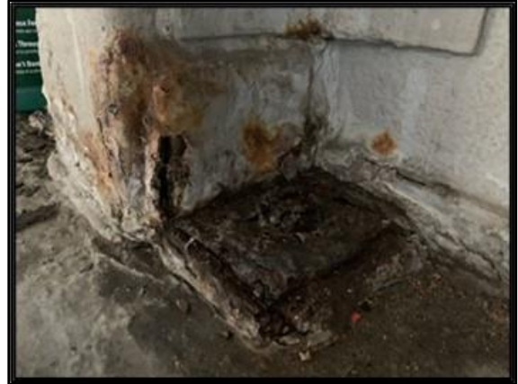
Figure 12: Observed Level 2 condition. Deteriorated angle and localized rusting observed on the HSS.
