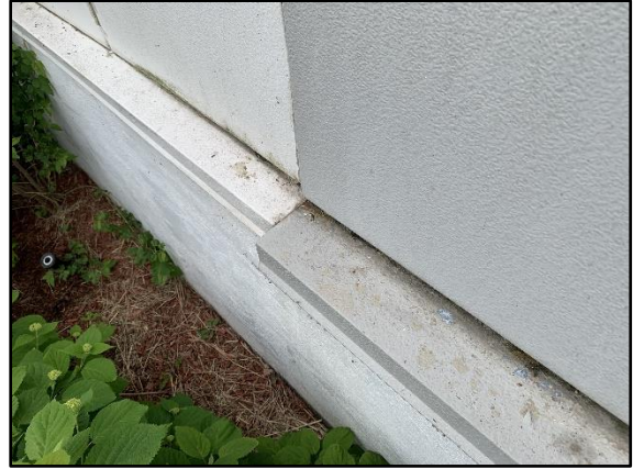
Figure 8: Noticeable plan offset between the concrete wall and metal panel on the exterior wall.
