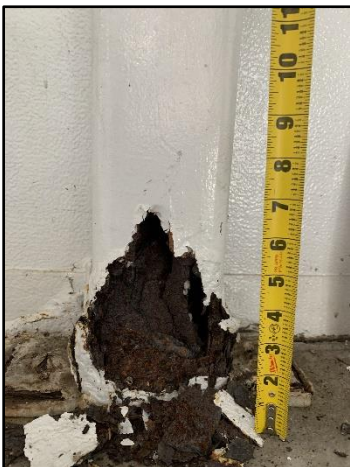
Figure 5: Significant deterioration of the angle and HSS section loss observed up to 7" high. (Level 3)
