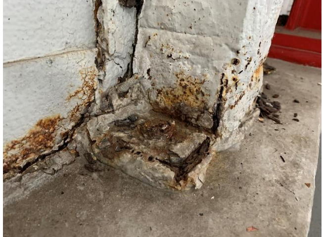
Figure 4: The angle shows slight deterioration and the HSS shows rusting. (Level 2)
