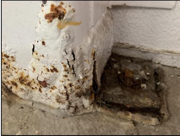
Figure 3. The angle shows deterioration and the HSS shows localized rusting. (Level 2)
