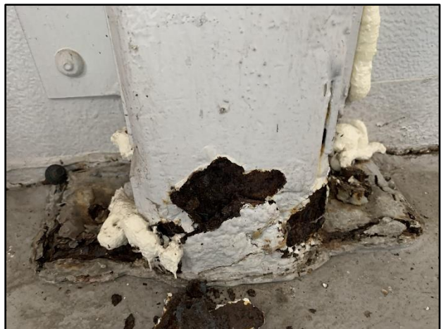
Figure 6: Significant deterioration of the angle and HSS section loss observed beginning above 3" from bottom. (Level 3)
