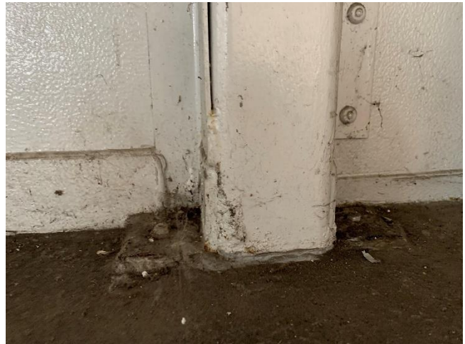
Figure 2: There is no visible deterioration on the HSS column. There is slight rusting on the angle. (Level 1)
