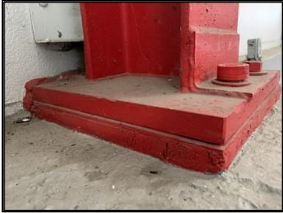
Figure 11: Base of a red painted steel column and base plate anchored to a concrete pier foundation in good condition.
